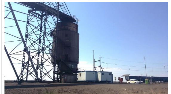
Rail load-out station with departing train
